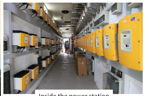
Inside the power station
