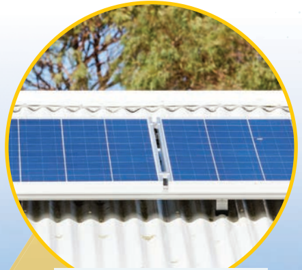
Solar panels on the roof of Bayswater School
