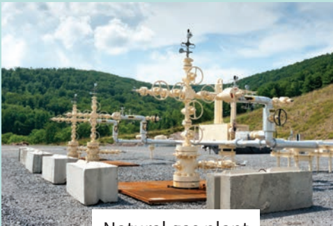
Natural gas plant
